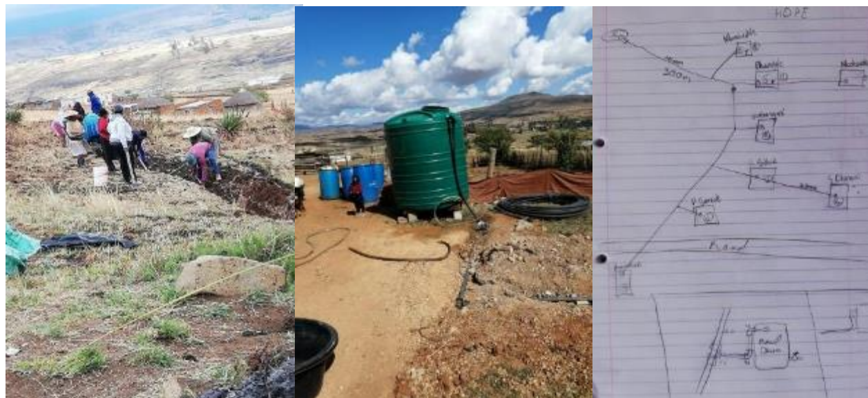
Figure 44: Left to Right; Digging the ditch from the spring to the header tank, the header tank at Phumelele Hlongwane's homestead – which was not installed on a level platform and has subsequently been corrected and an initial rough layout drawing of the flow of the water to participants' homesteads.
