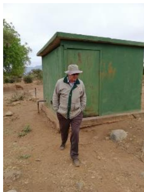
Figure 50: The municipal pump station, not in use, but which participants thought provided an example of the kind of “protection” they would like for their borehole. It was explained by the facilitation team that such a structure is costly and was not budgeted for.
