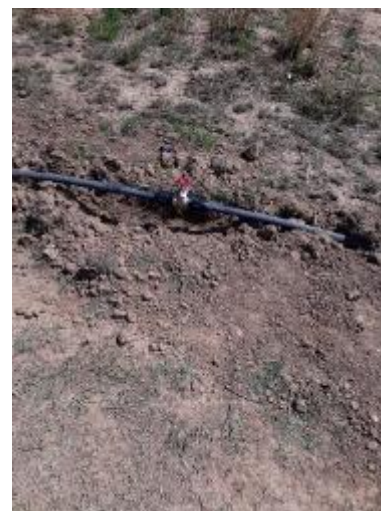
Figure 48: The main valve in the pipe-line shutting of water from the header tank
