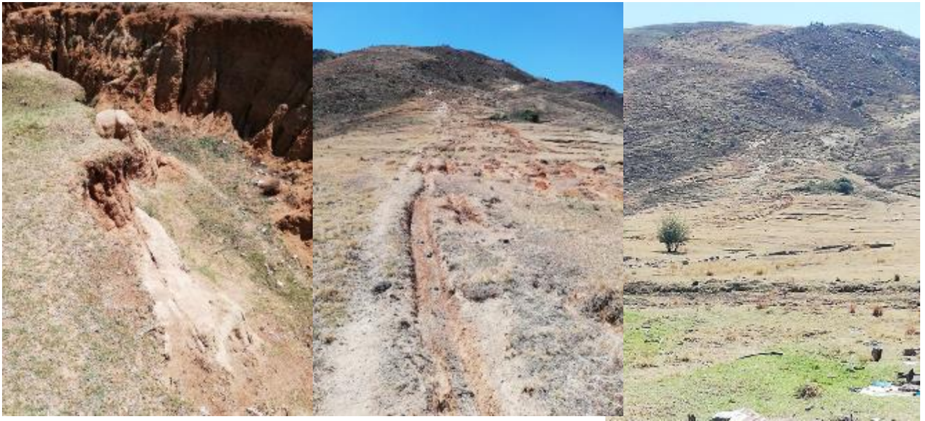
Figure 70: Left: The large donga separating the two sides of the village. Centre: Erosion due to cattle movement and overgrazing. Right: burning of the mountain for early spring grazing, also leading to erosion.
