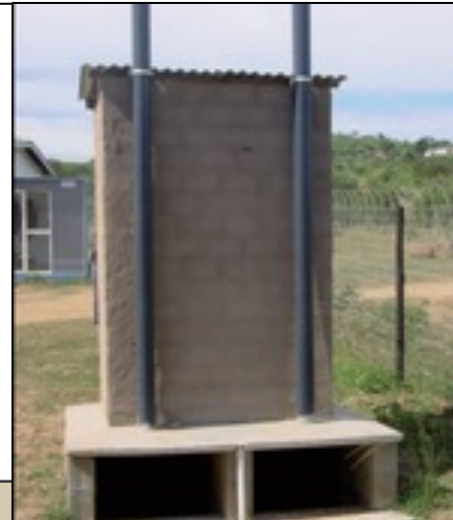
USDDTs: Urine diversion dehydration toilets (>10 years, empty at annual intervals)
