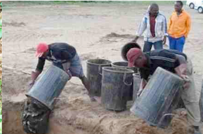
Entrenchment of faecal sludge and planting of trees
