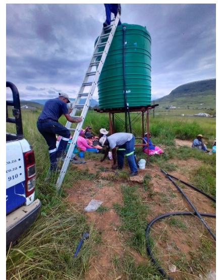
Figure 9: Above Left to Right: the Pump connection, attached to Mrs Fiansi Mpulo's homestead electricity supply, the 5000l header tank with tap and the top 2500l header tank with tap.
