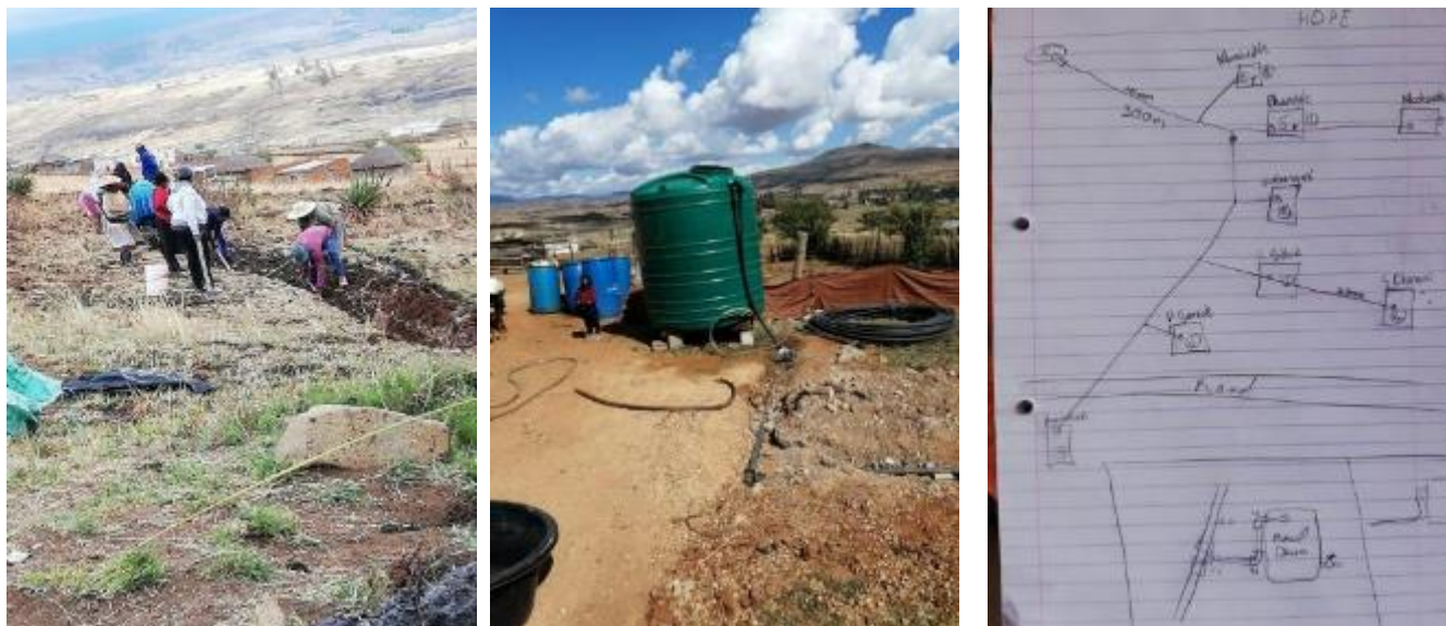
Figure 19: Left to right: Group members digging the ditch from the spring to the header tank. The header tank at Phumelele Hlongwane's homestead – which was not installed on a level platform and has subsequently been corrected. Initial rough layout drawing of the flow of the water to participants' homesteads.
