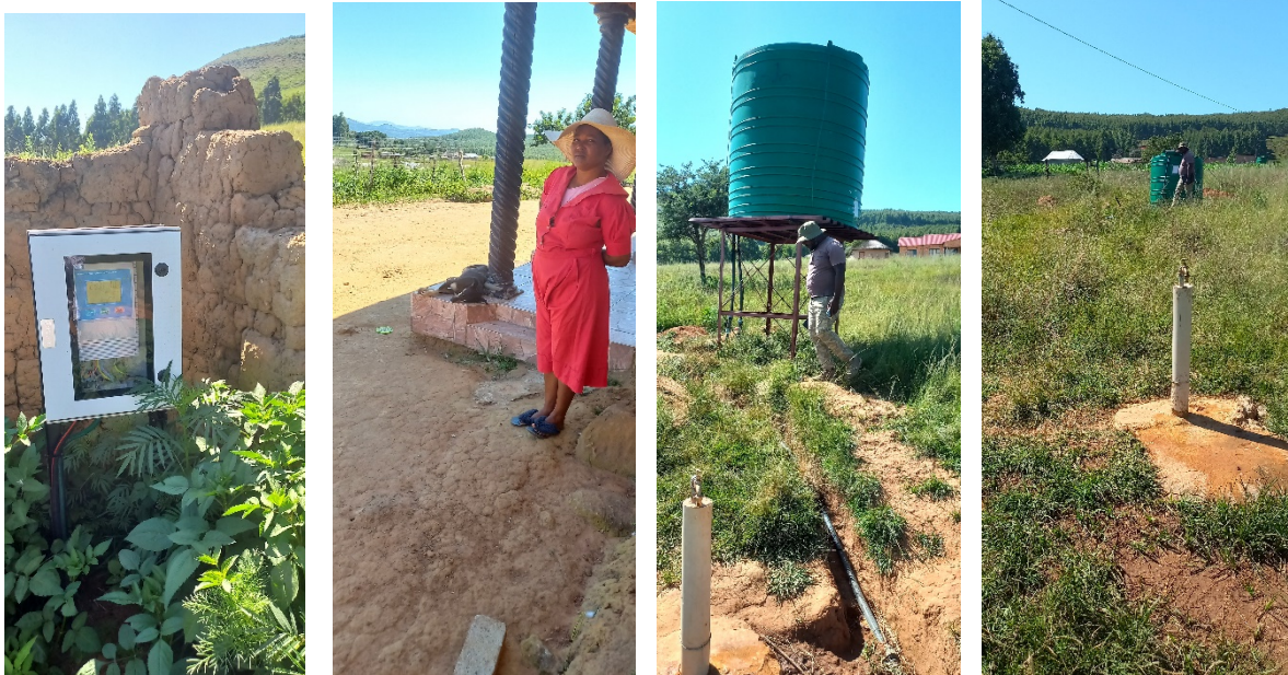
Figure 9: Above Left to Right: the Pump connection, attached to Mrs Fiansi Mpulo's homestead electricity supply, the 5000l header tank with tap and the top 2500l header tank with tap.
