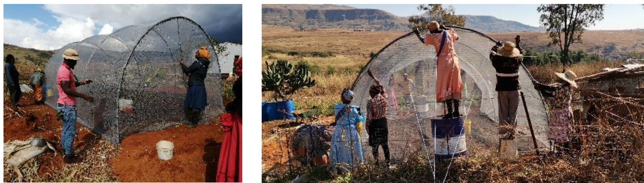
Figure 10: Above Left and Right- Final sewing of the panels onto the arches and putting up the string and Y-standard anchors for the tunnels as two different households. Not that the beds are planted to seedlings on the same day.
