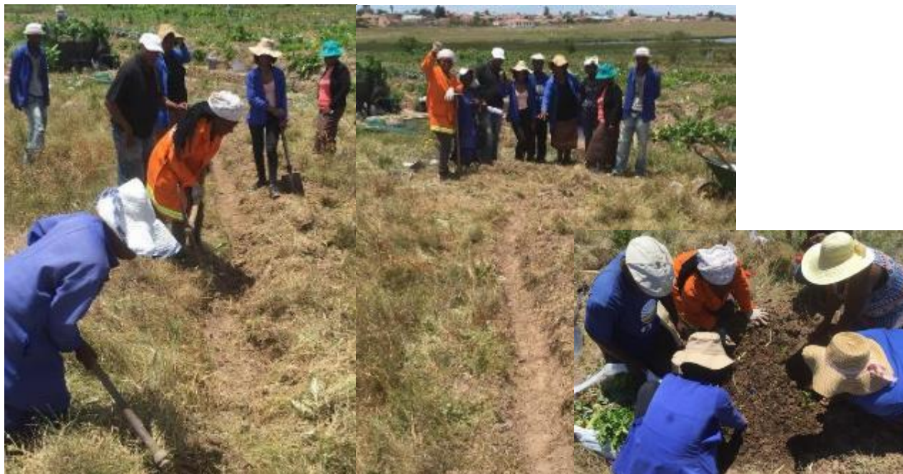
Above Left to Right; diversion furrow and infiltration pit implementation process
