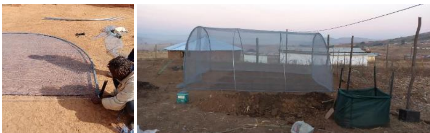
FIGURE 18 : ABOVE LEFT: BENDING OF PIPES, CUTTING AND SEWING OF NETTING ONTO THE ARCHES FOR ABOVE RIGHT: CONSTRUCTION OF A DEMONSTRATION TUNNEL IN CENTOCOW
