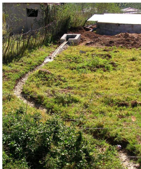
Figure 7.1 Diversion furrow leading to a catchpit
