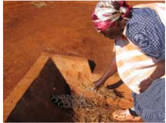
You should clean debris out of the strainer in your silt trap after each storm
