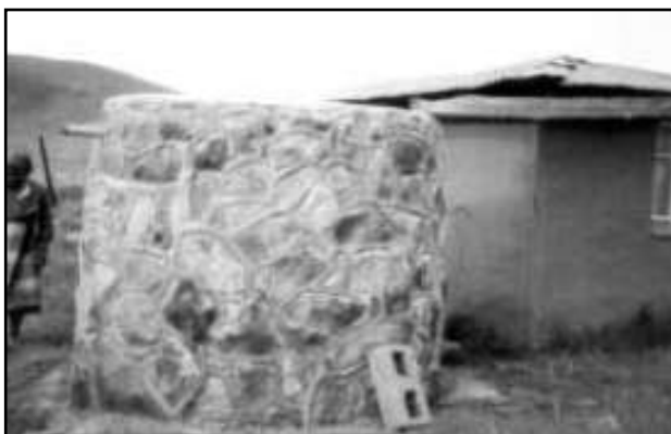
Roof tank built from stone and cement
