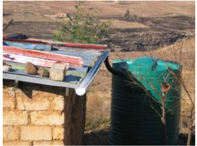
Gutters should be placed as close to the roofline as possible so that most rainwater will go into the tank.
