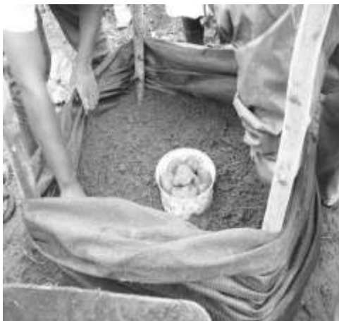
Participants in Potshini are busy filling up the stone column in the middle. Note the small white bucket (bottomless) that help to provide a rigid structure for the placing of the stones.
