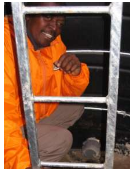
Be careful not to damage the non-return valve at the bottom of your tanks when you are cleaning them.
